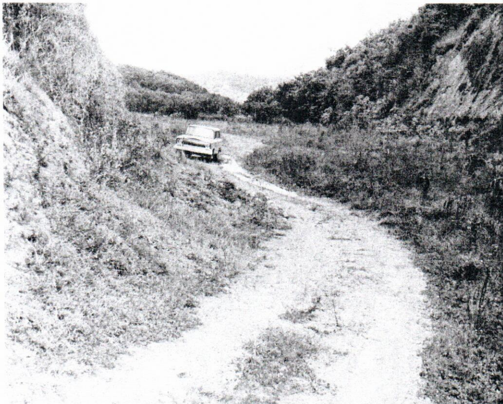
EMERGENCY SPILLWAY OF LAKE CARITE SHOWING SMALL SWAMP CONTAINING BIOMPHALARIA GLABRATA JULY 1976
