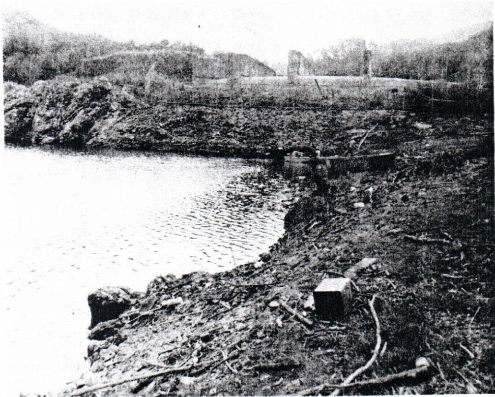
SPILLWAY OF LAKE GARZAS
