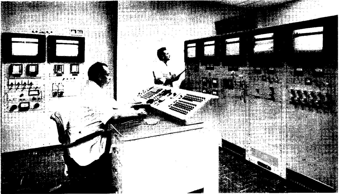
CONTROL ROOM FOR P.R.N.C. POOL TYPE RESEARCH REACTOR DESIGNED FOR OPERATION AT A 5 MEGAWATT POWER LEVEL
