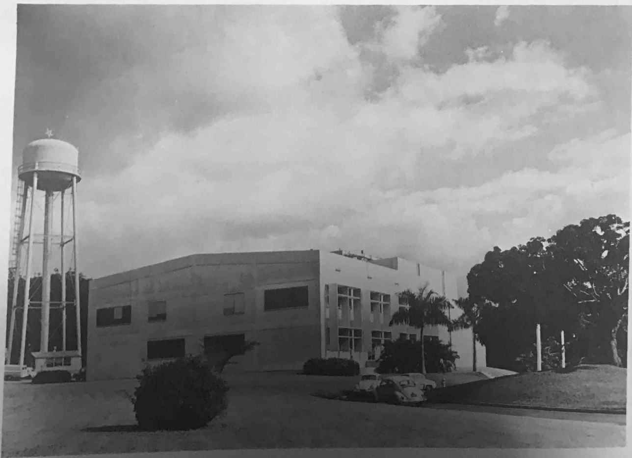
PRNC's main installations in Río Piedras (top) and Mayaguez (bottom).
