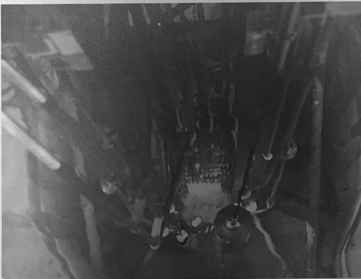
View from reactor bridge, looking down at TRIGA reactor core.
