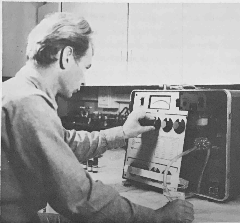
Dr. Seppo Kolehmainen determining salinity of sea water with induction salinometer.
