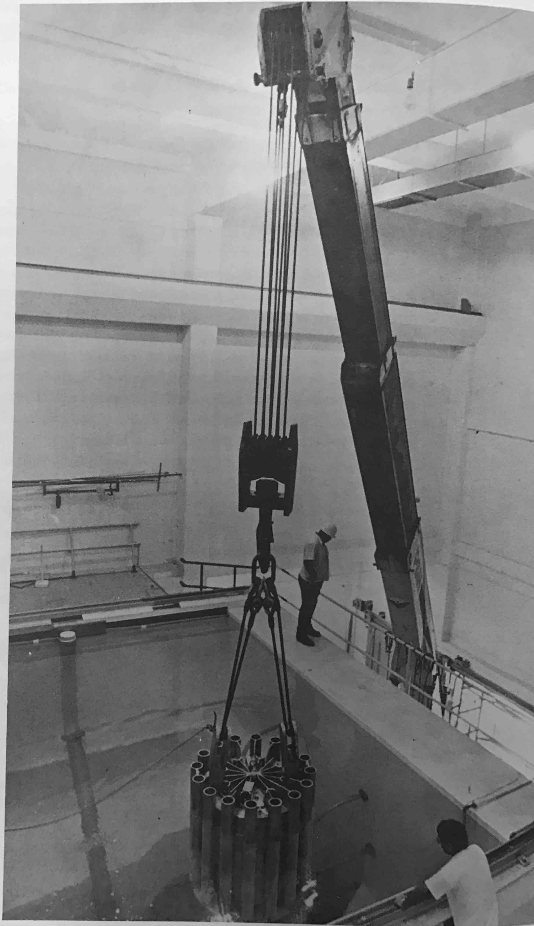
Richard Brown Campos Head of Reactor Operations, supervises the removal of spent fuel rods from the TRIGA-FLIP reactor.
