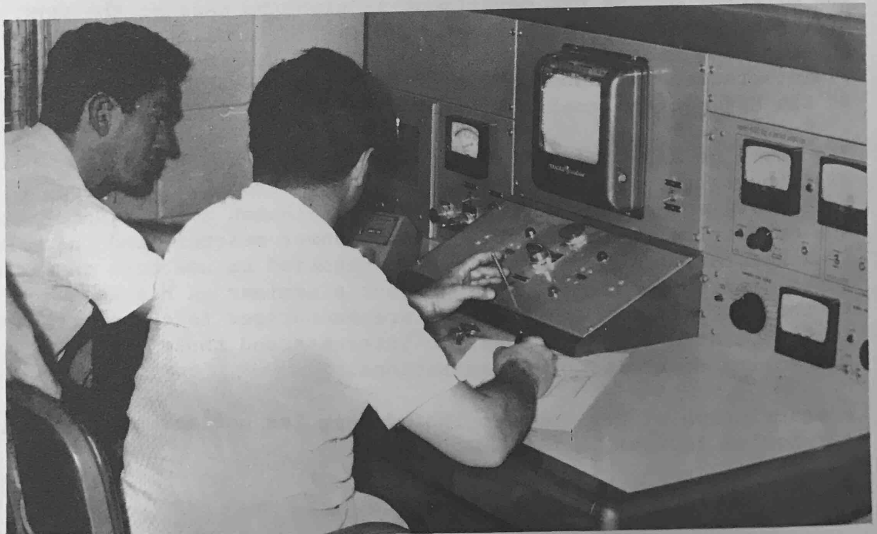
Figure 1. A graduate student observing the control console of the L-77 homogenous reactor with a reactor operator.
